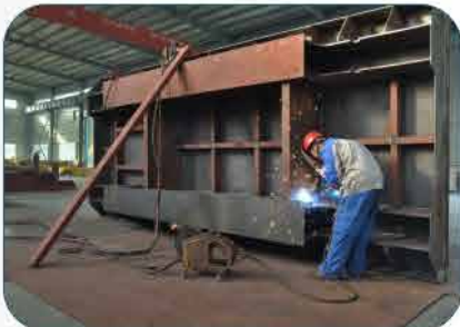
箱梁式结构 Box beam type structure
