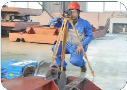
平整度测量 Measuring flatness
